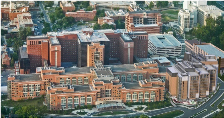
Looking from north to south
